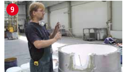
Before external heating, venting holes are pierced into the INSURAL 10 refractory layer
