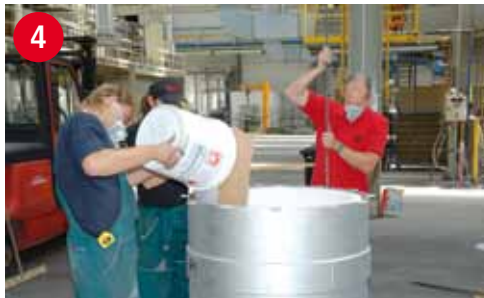
Filling the gap between steel shell and ATL with INSURAL 10 material
