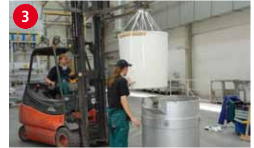
Inserting ATL lining in the steel shell
