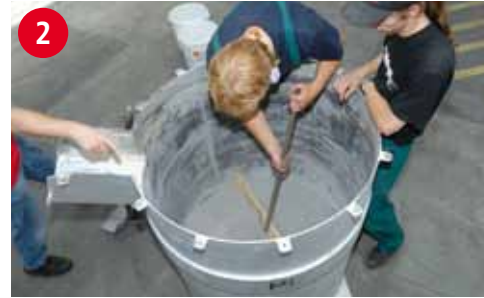
Levelling of INSURAL 10 material at the bottom of the ladle
