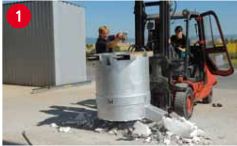
Easy removal of old lining
