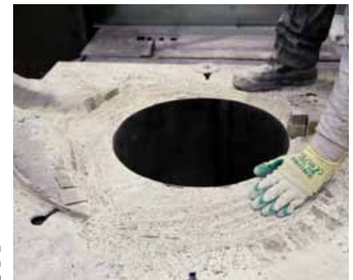
Coreless induction furnace lined with KELLUNDITE 400
